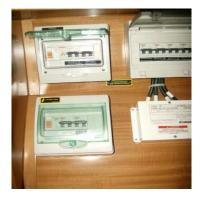
Located to the right of the entrance to the starboard aft cabin are the main breakers for the air conditioning units and 12v systems.
