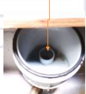
Fit dinghy pump nozzle and force the blockage out
