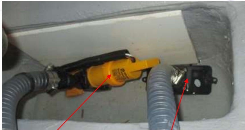
Automatic bilge pump
