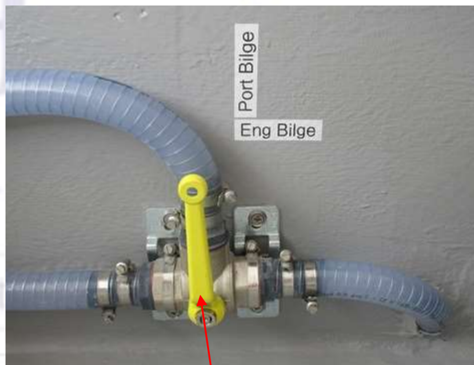
Manual bilge pump diverter valve in cockpit lockers
