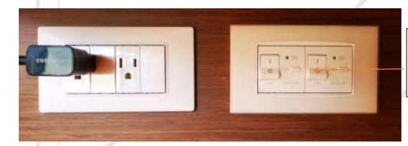
GFCI switches are below 12-Volt panel. If there is no power coming from your outlets, ensure these switches are in the on
