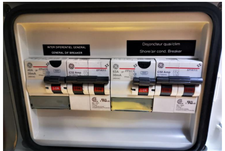
Generator/Shore Power Breakers Behind Generator
