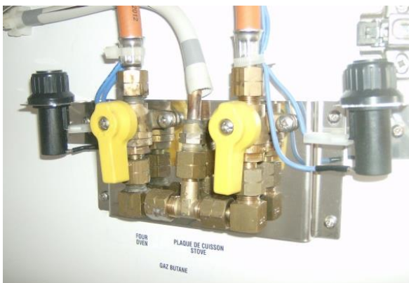
PROPANE SHUT OFF VALVES BELOW GALLEY SINK
