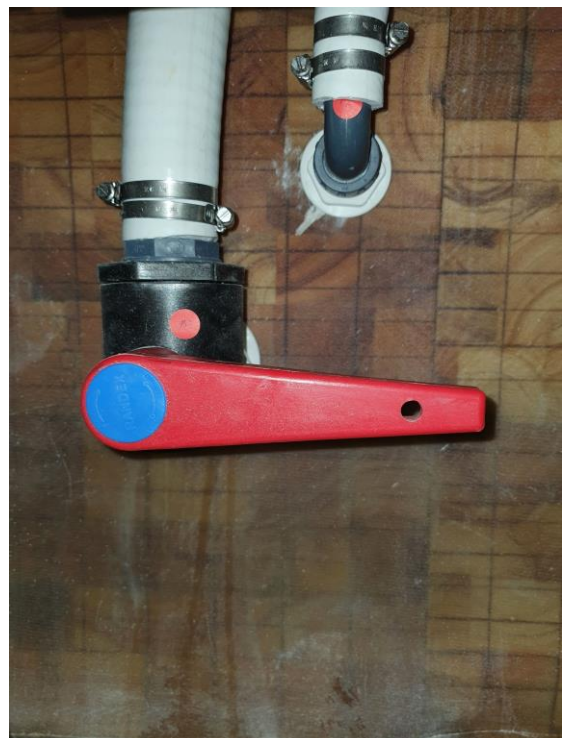
Hold Tank Evacuation Valve (Closed Position)
