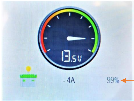
Domestic/House battery voltage
