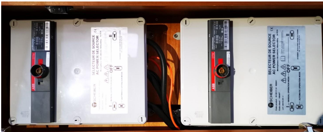
Selector Switches and removable handles in starboard aft cabin locker.
