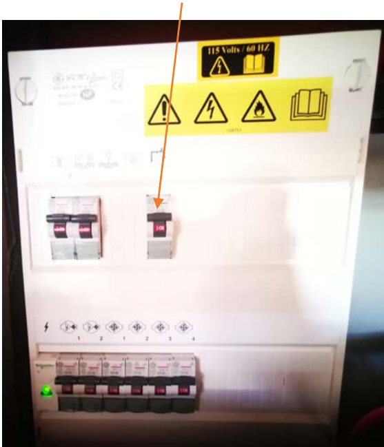
Ice maker breaker (locker above 12V panel)
