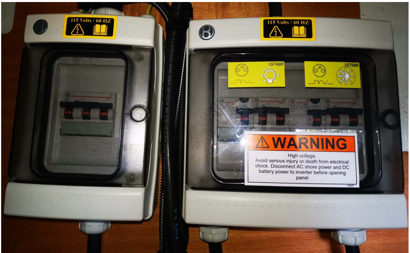
Generator/Shore power breakers in starboard lazarette
