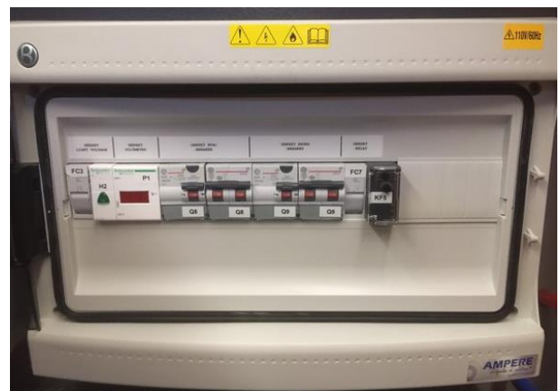
110V Breakers under stbd aft cabin bunk (remove mattress for access)
